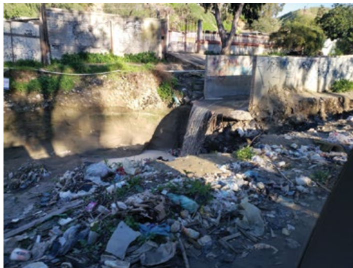
Figure 2. Example of unarmored channel contributing to excess cross-border sediment and trash.
