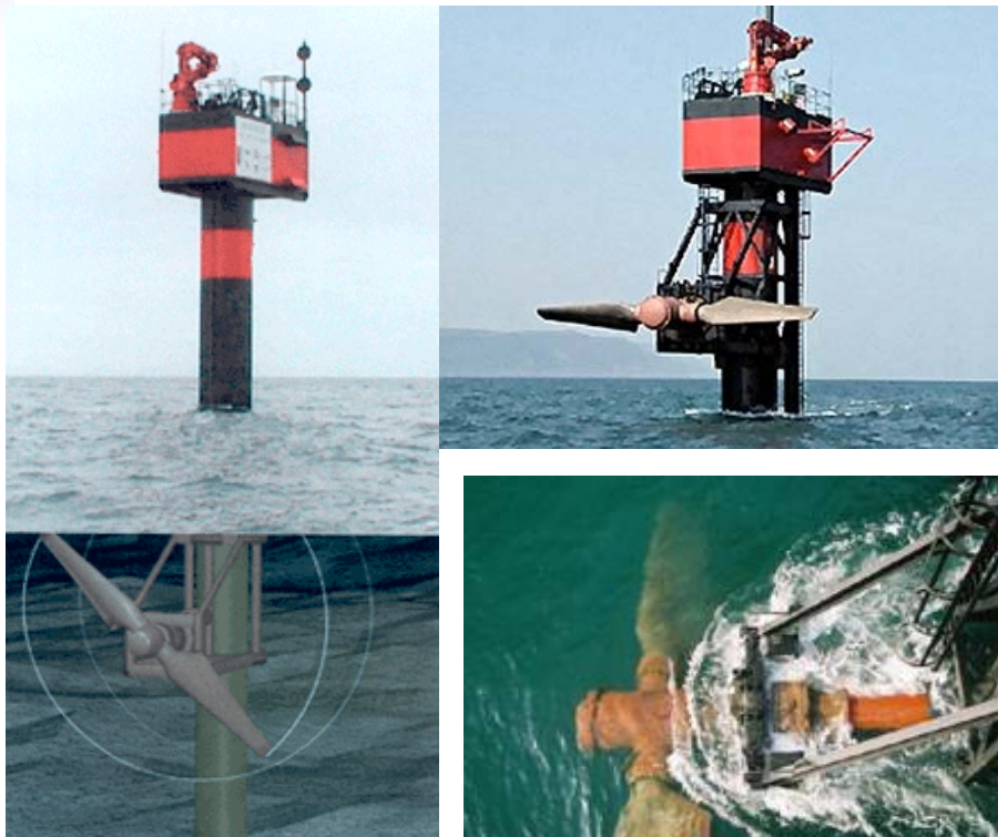
SeaFlow experimental 300 kW prototype (11-m rotor diameter) operating in Bristol Channel since May 2003; not connected to grid)
